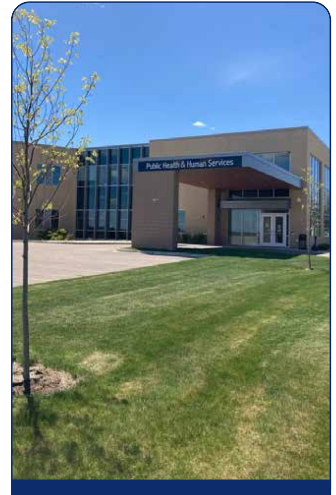
Green County Government Services Building
